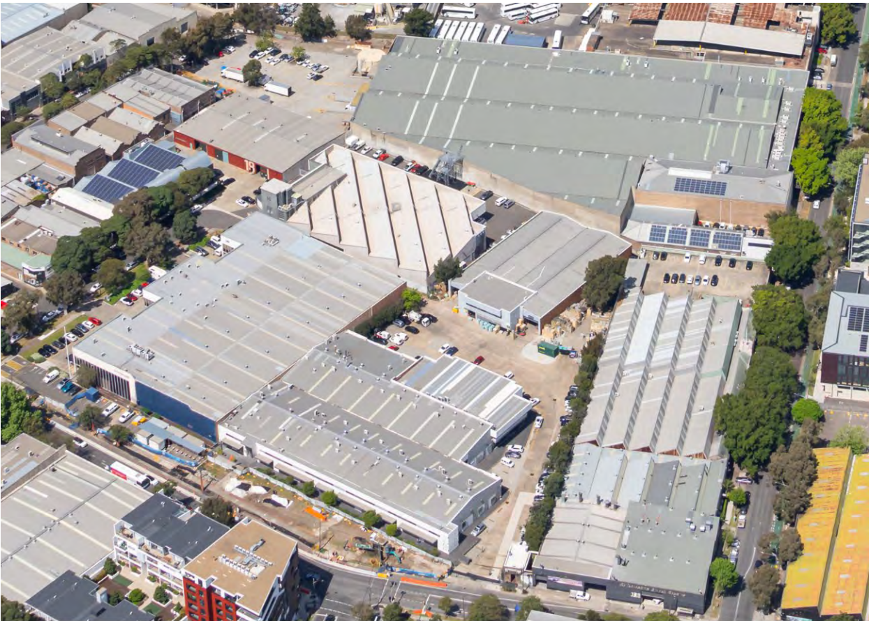
Figure 5: Larger warehouse buildings on corner of McEvoy and Bowden Streets
